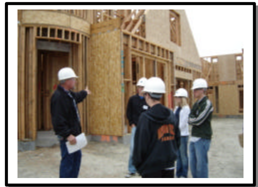
A tour was given of all aspects of the construction process.
