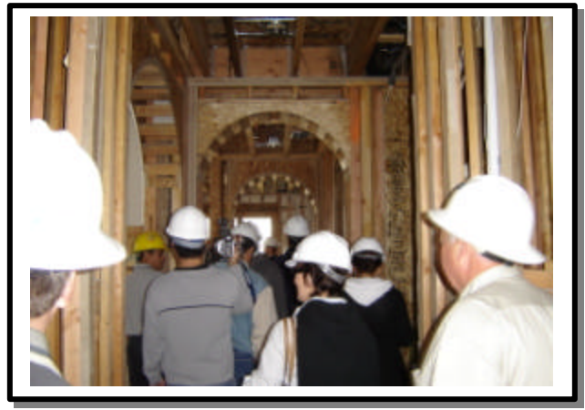
Each phase of construction was explored inside and out.
